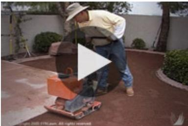
Areas that are bordered by sidewalks, concrete or other defined space require special care. Like the other compaction methods mentioned, start with the perimeter. Working with caution, guide the plate compactor slowly around the defined border. Be aware of your surroundings and work to not run into the concrete or border.
