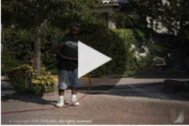
The last step in building your sub base is to wet down the aggregate. This creates a harder top layer for your base. Sometimes, it's a good idea to compact the base with the plate compactor and hand tamp one final time. If you do re-compact the base, you will may need to spray it down again before proceeding.
