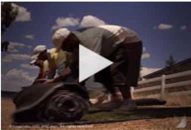
After you have measured and marked your sections, roll the turf over the base and cut each section. It is a good idea to leave a little extra length while you trim and position the turf. You will trim off the extra length once you have all the turf in position and are ready to cut the final shape.
