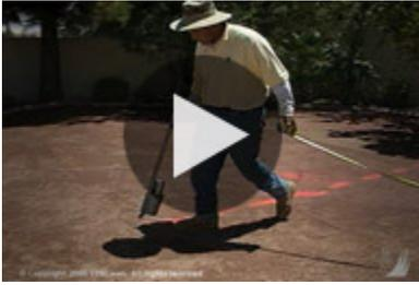
Before you cut a single piece of turf plan your cuts by measuring and marking on your base. This will help you determine the section sizes of the turf and determine seam locations. It is recommended that you make your general size cuts somewhere other than on your base, like a driveway or other large flat surface, before laying them into position.
