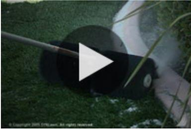
Using a power broom to work the infill down into the fibers is a quicker, more efficient method. Not only does it speed the process along, it helps disperse both sand and rubber evenly throughout the lawn. It also defibrillates or breaks up the polyethylene fibers to create various blade widths for a more natural appearance.
