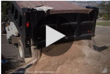
When having aggregate delivered to the job site, try to have the load placed as close to the installation area as possible. Always check aggregate before having it dumped to make sure it is the correct rock size and verify your order. You don't want to have to return the aggregate once it has been dumped onto your property. You will need crushed aggregate that has a 1/4-inch to 3/8-inch minus rock size to build the proper base.
