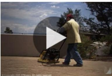
Using a plate compactor start the compaction process with the outside perimeter. Compact around the perimeter 3-4 times moving inward with each pass before working your way through the inside of the installation area.
