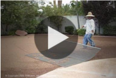
As an optional final step in compacting the sub base, use a screen or drag rake over the entire area. This helps level any inconsistencies on the base surface and removes larger rocks and debris.
