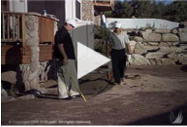
In preparing for synthetic turf installation preliminary measurements are made to define the area for installation. While taking measurements, use spray paint to determine final shape of your lawn. You will need to take into account how the grass will border against other landscape elements and you will need to make sure you have enough material for the project.
