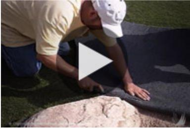
Cutting around rocks or other odd-shapes requires many small cuts to position the turf properly. Be sure to plan each cut and only remove as much turf that is absolutely necessary. Take your time and don't try to remove large sections of turf all at once.
