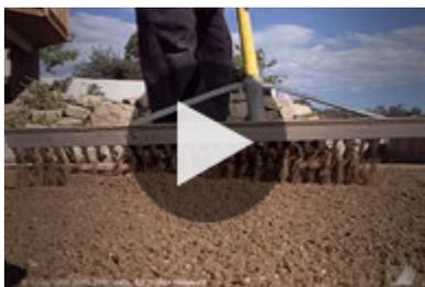
Spreading aggregate over the installation area is the first step in creating your sub base for SYNLawn. When complete, the sub base will be a hard, smooth surface for the turf to lie over. The sub base gives the turf a solid foundation while providing proper drainage dispersion.
