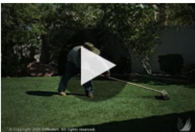
Brooming the rubber grinds is a required step to work the infill down into the fibers of the turf. It also helps disperse the infill and even out the high spots created during the application of the rubber grinds.
