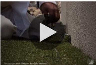
When cutting along the side of a wall or similar structure, keep the turf snug up against the wall edge. Always try to cut from the backside of the turf whenever possible. If cutting from the top side use caution to not cut away too many fibers.
