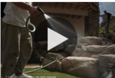
The final step of the infill process is wetting down the turf with a garden hose. This helps drop the infill material down into the fibers and to the base. It also helps clean excess dust and debris left behind during the infill process.
