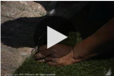
Using yard staples is a recommended method of securing the turf edges around the perimeter of the installation area. Yard staples are generally found at landscape nurseries or home improvement stores in the landscaping section.
